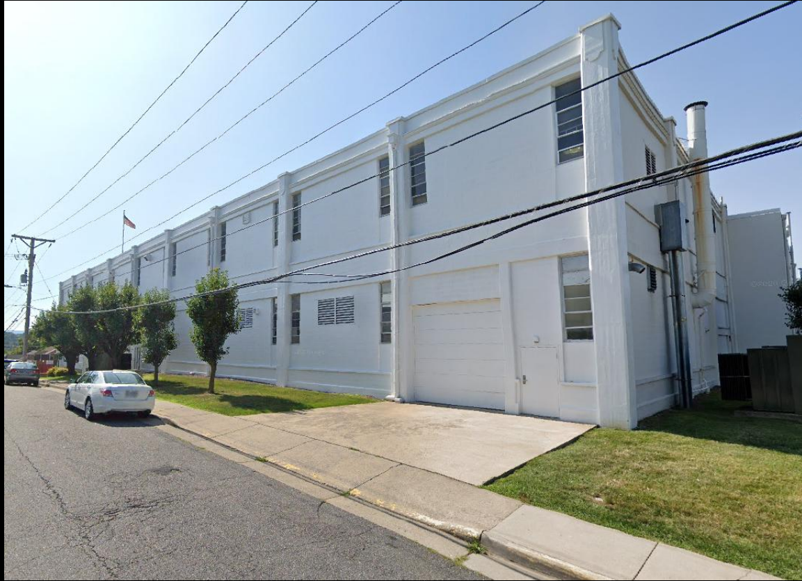
Northern portion of the building, adjacent to West Wolfe Street
