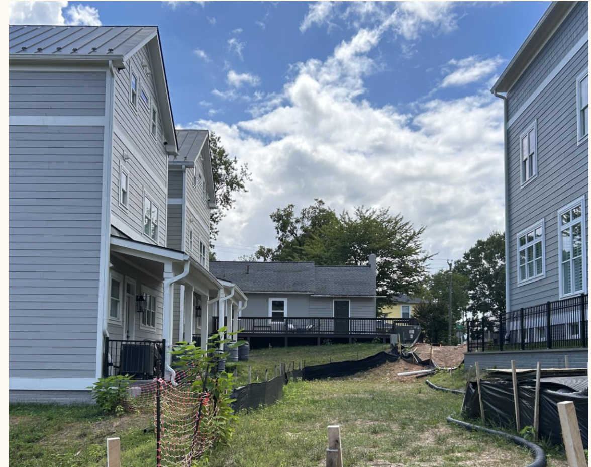
Infill development example in Charlottesville (Grove Street). Rain barrels and future green roofs over the porches (left side) and permeable paver driveways are being used to meet some stormwater management requirements onsite
