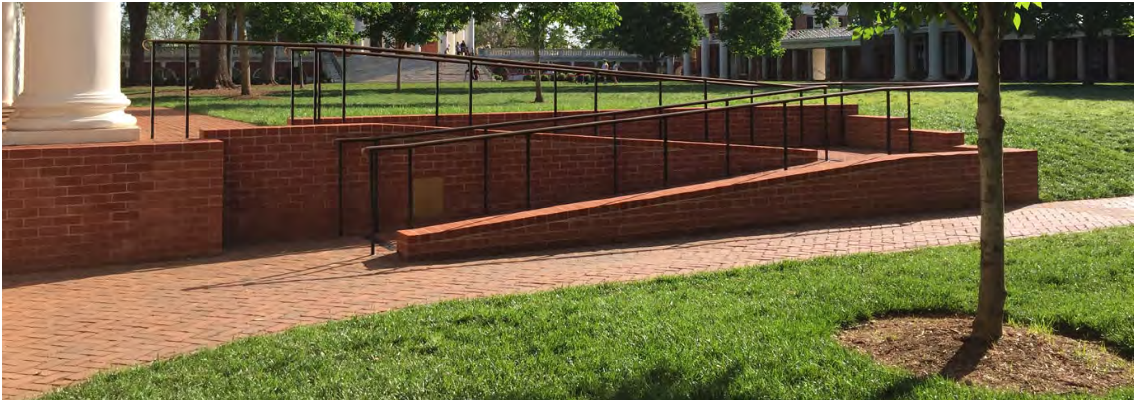
BRICK RAMP AND ORNAMENTAL METAL HANDRAIL
