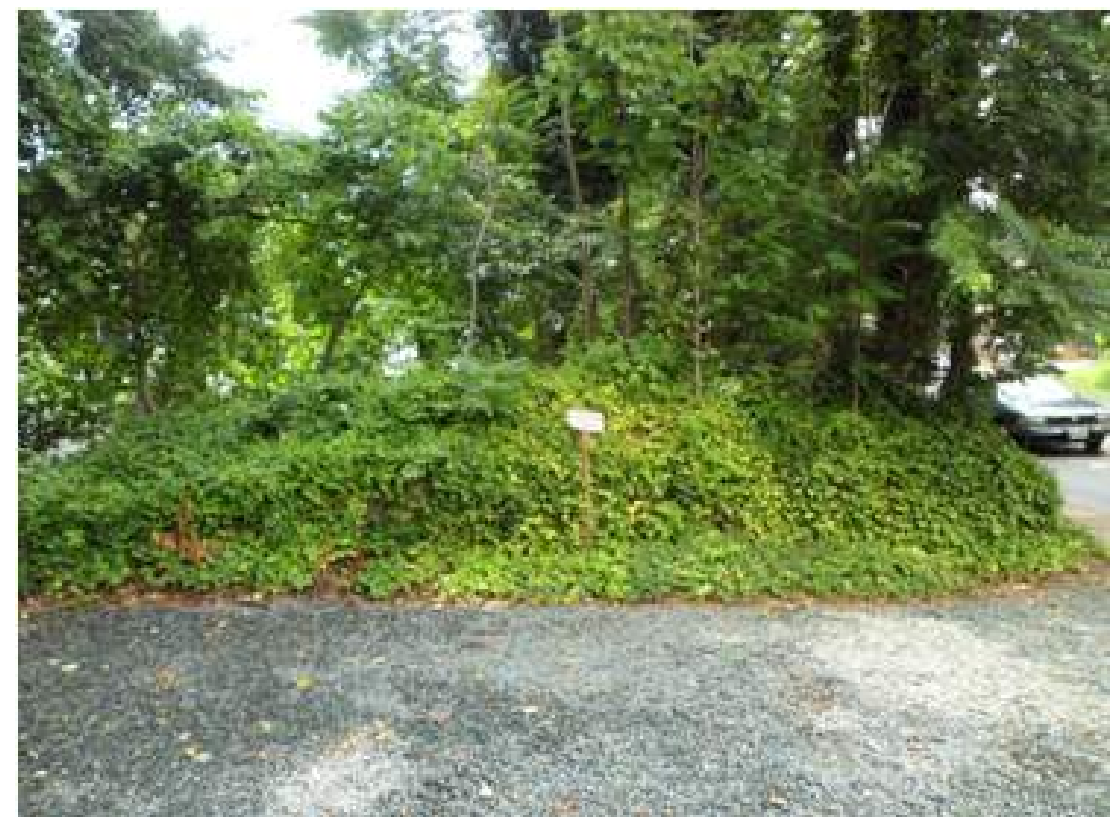
VIEW OF GARAGE FOUNDATION
