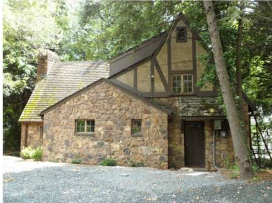
VIEW FROM EMMET STREET S
