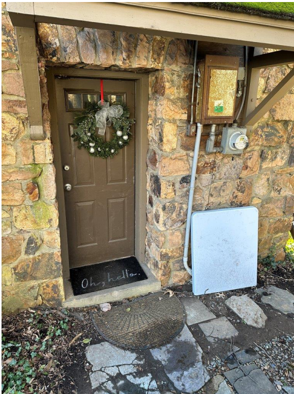
New front door w/ bracketed roof
