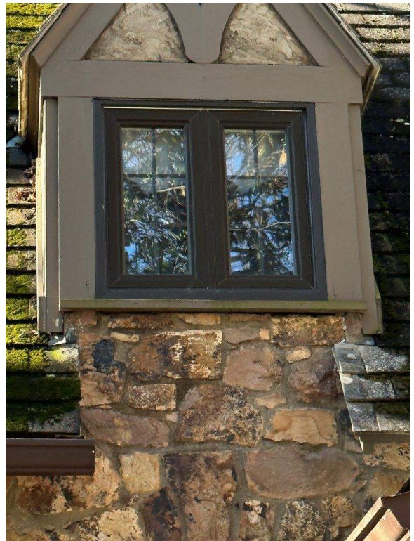
Dormer showing all materials present
