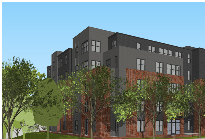
rear corner along Observatory Ave.
