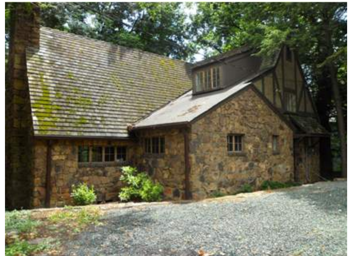
VIEW FROM EMMET STREET S
