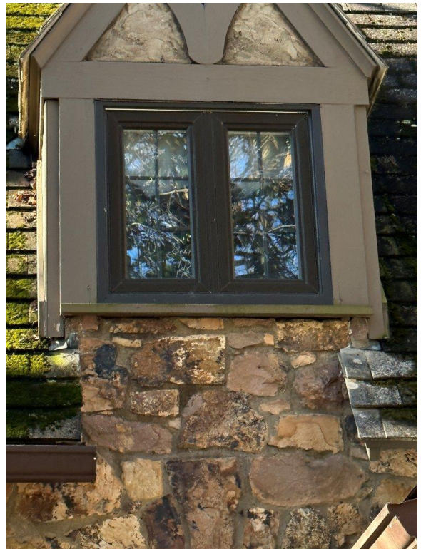
Dormer showing all materials present
