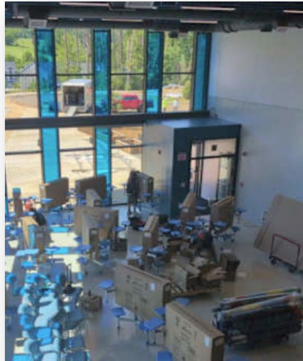
Mountain View Upper Elementary Construction
