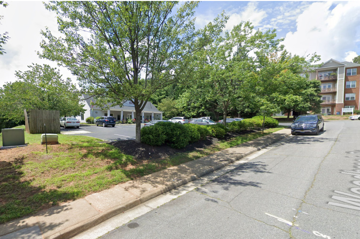
Image 7 - Subject site and adjacent apartment complex
